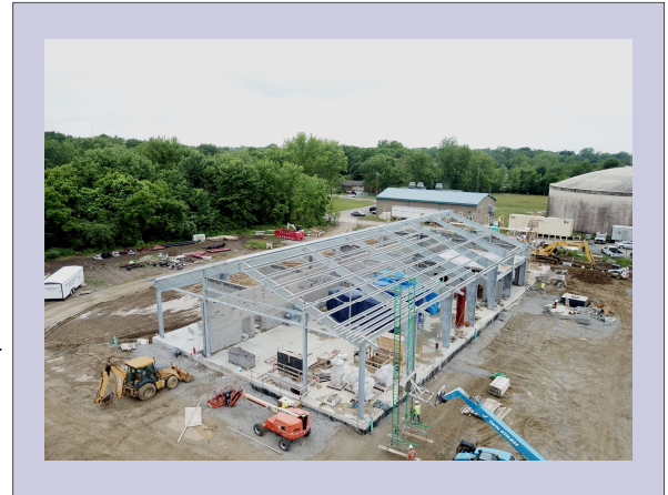
NF Building Construction — June 2021
