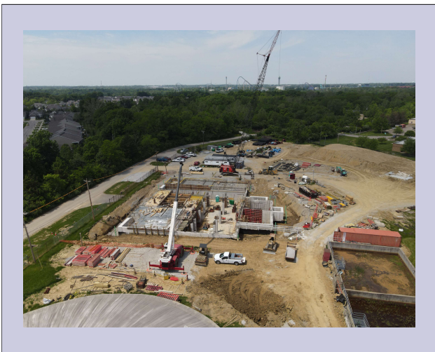
NF Building Construction — May 2021
