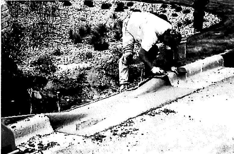
Figure 31: image of retrofit curb cut
