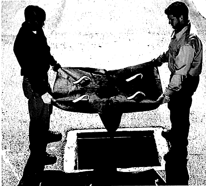
Figure 29: example of catch basin (storm drain) insert
