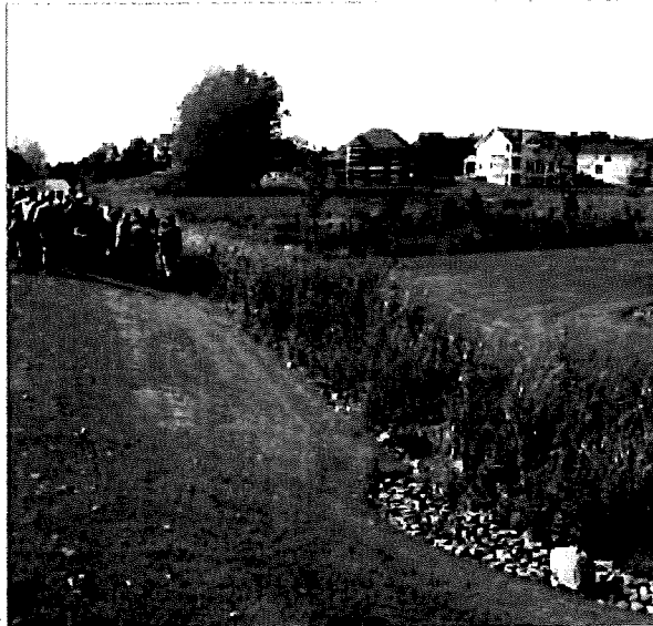
Figure 33: image of vegetative swale in residential district
